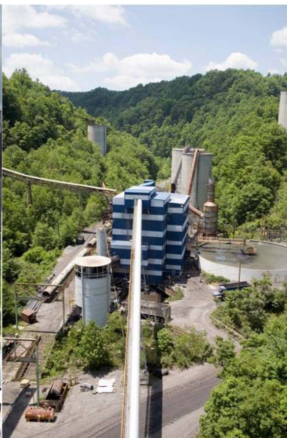
> Gauley Eagle preparation plant and infrastructure
